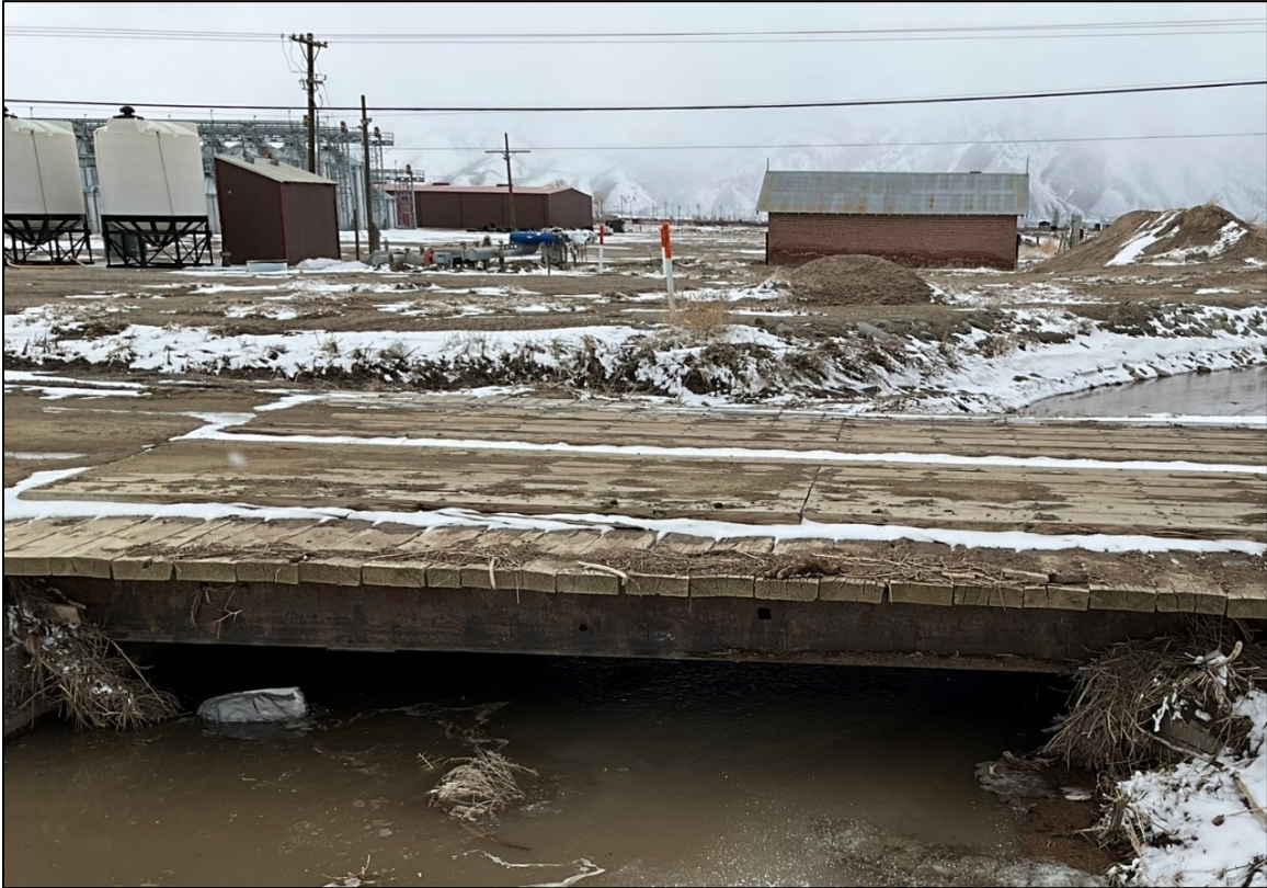
Figure 6-10. Heybourne Road Private Bridge
