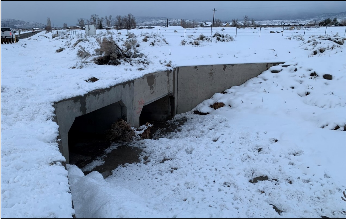
Figure 6-9. East Valley Road Box Culvert
