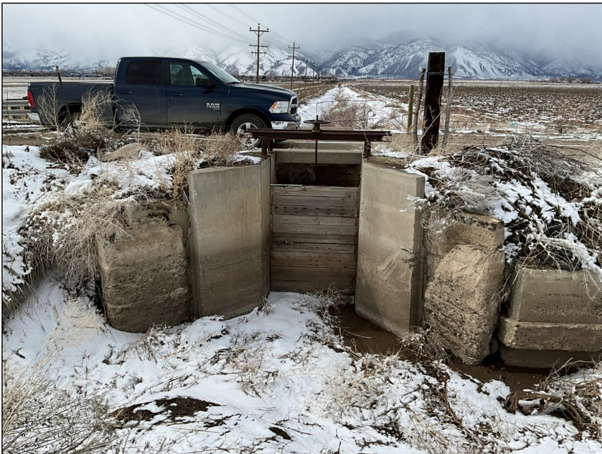
Figure 2-1. Example of Typical Structure Observed in the Field
